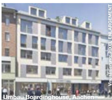
Umbau Boardinghouse, Aachen
